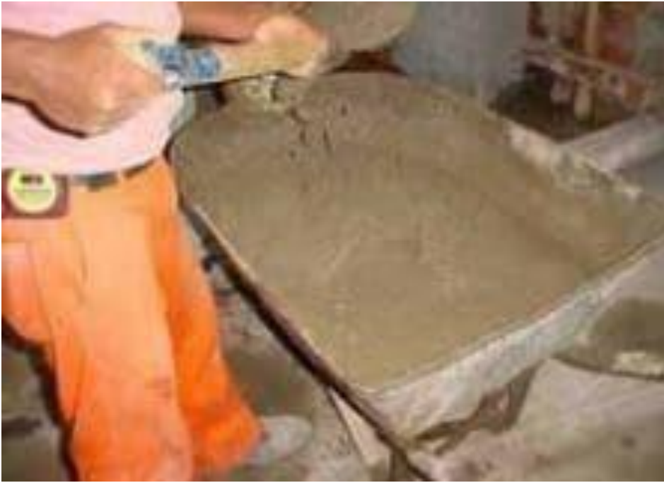
Fig. 5: Mortar Preparation
