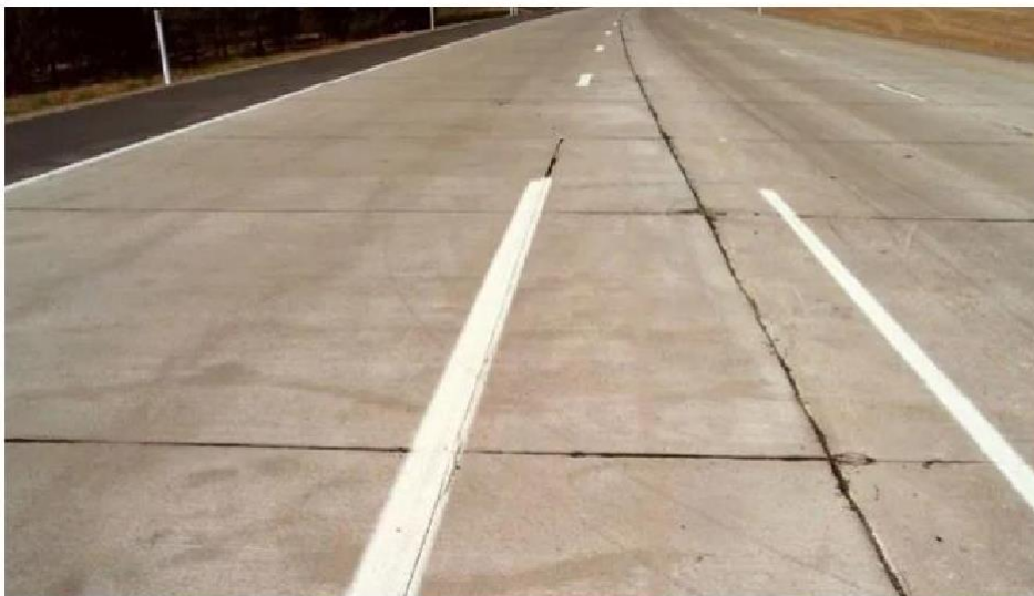
Contraction Joint in Concrete
