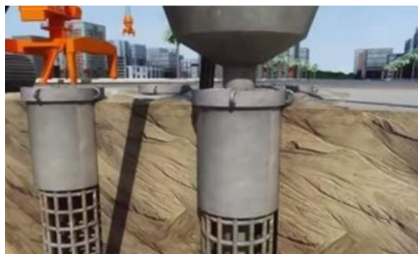
Fig.4. Diaphragm Joints by Disposable PVC Pipes
