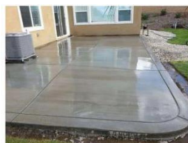
Decorative Concrete Joints
