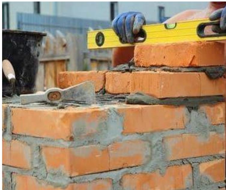
Fig. 8: Checking level of brick masonry
