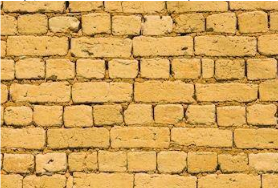
Fig. 1: Brick work in mud
