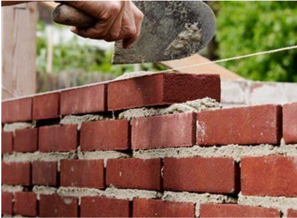
Fig. 2: Brick work in cement
