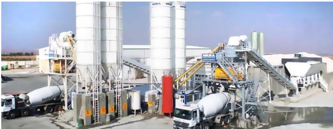
Fig: Stationary Concrete Plant
