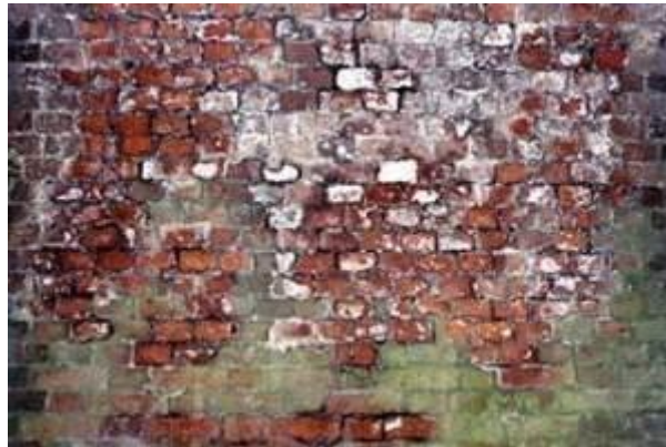
Test for efflorescence.
